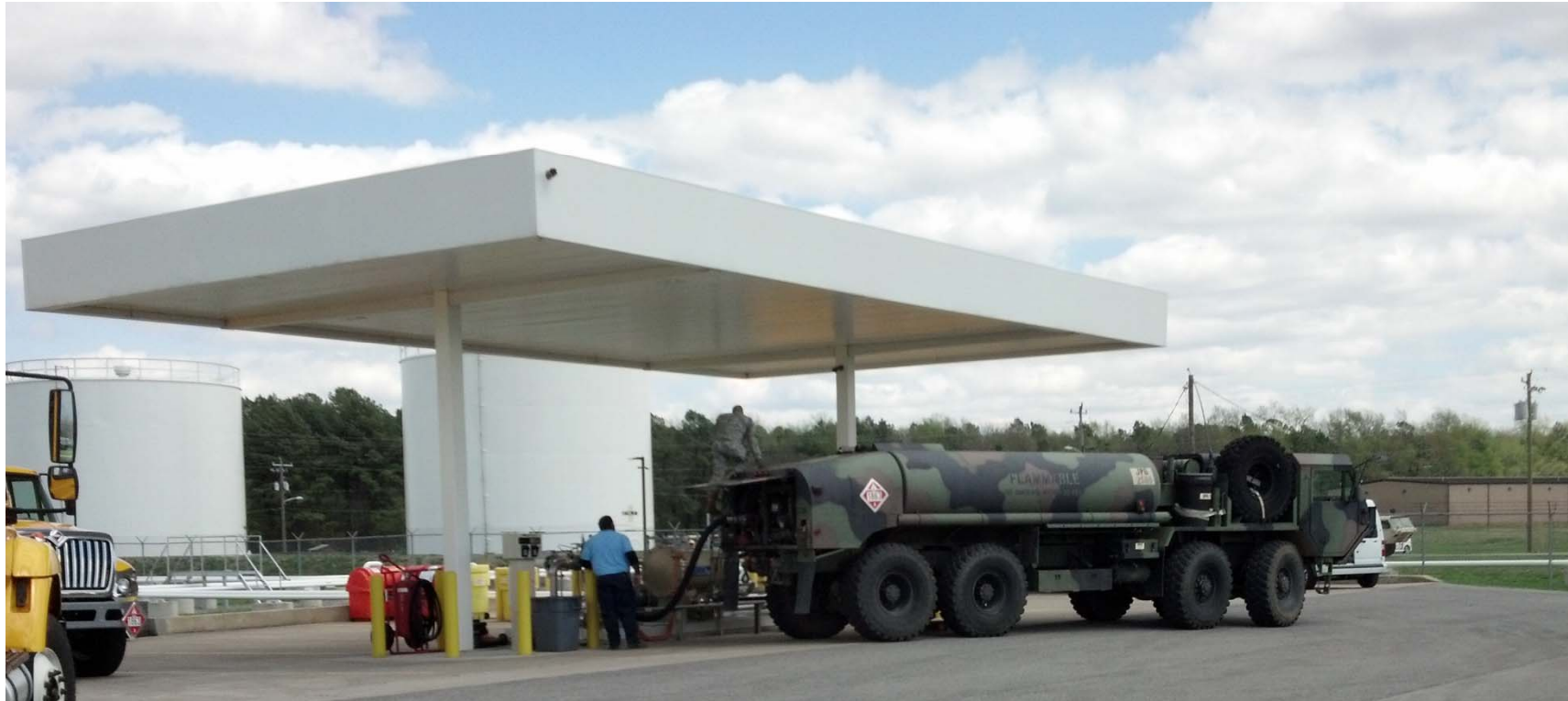
Dispensing Station for Refueling Trucks
