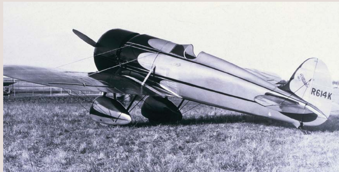
Rear, quarter-view of R614K parked at Travel Air Field before it was flown to Cleveland for the National Air Races. The windshield had been enlarged from the original design to provide more protection for the pilot. (Kenneth D. Wilson)
