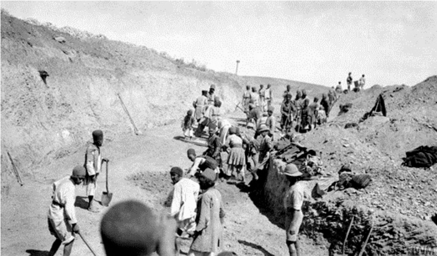
Figure 9. Persian laborers constructing a road through the Asadabad Pass under the supervision of the British Army 'Dunsterforce'.
