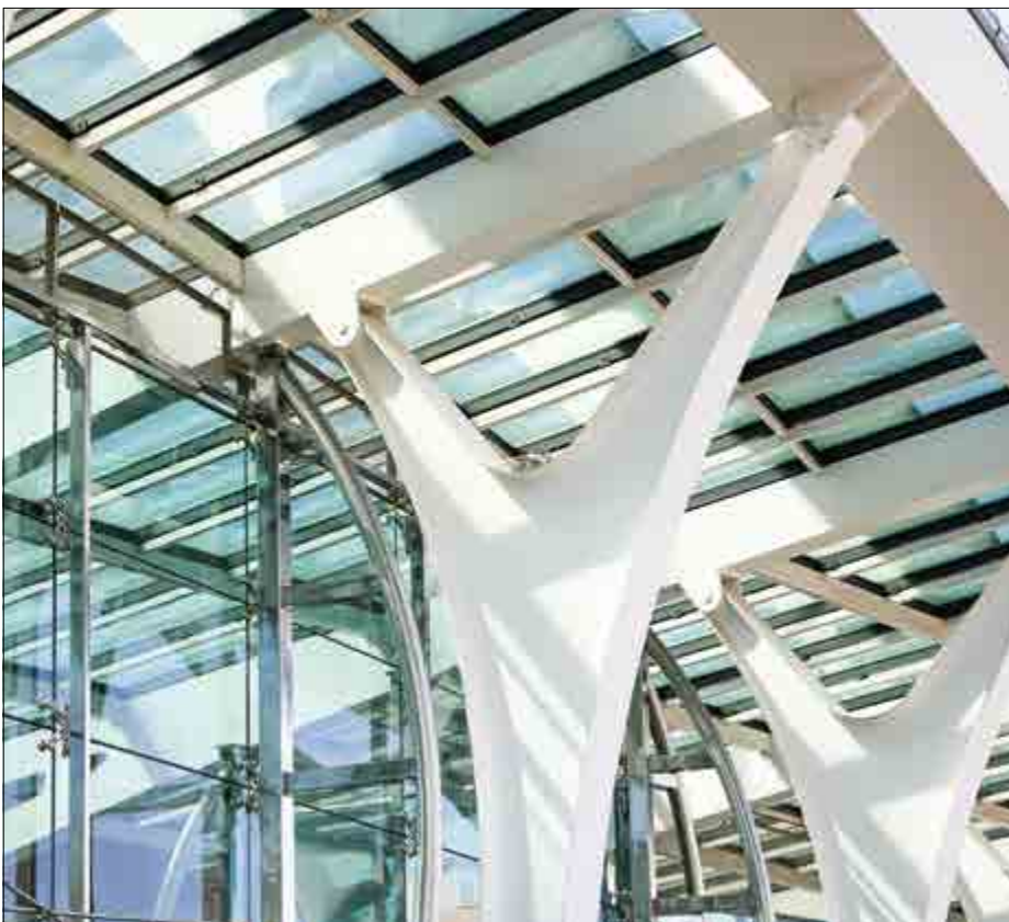
Figure 22 Sloped Overhead Glazing Source: Shutterstock
