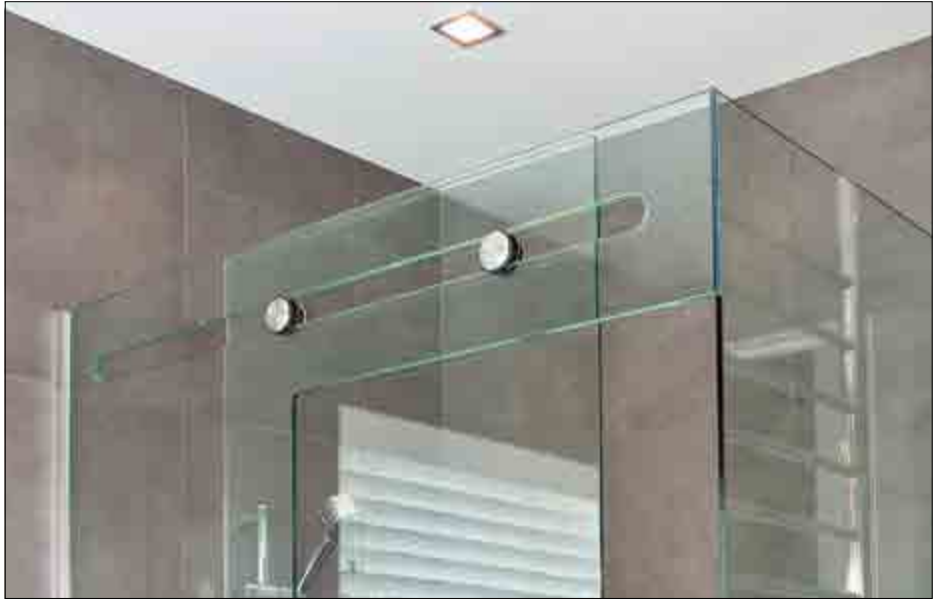
Figure 51 Edgework and Cut Outs in a Shower Screen
