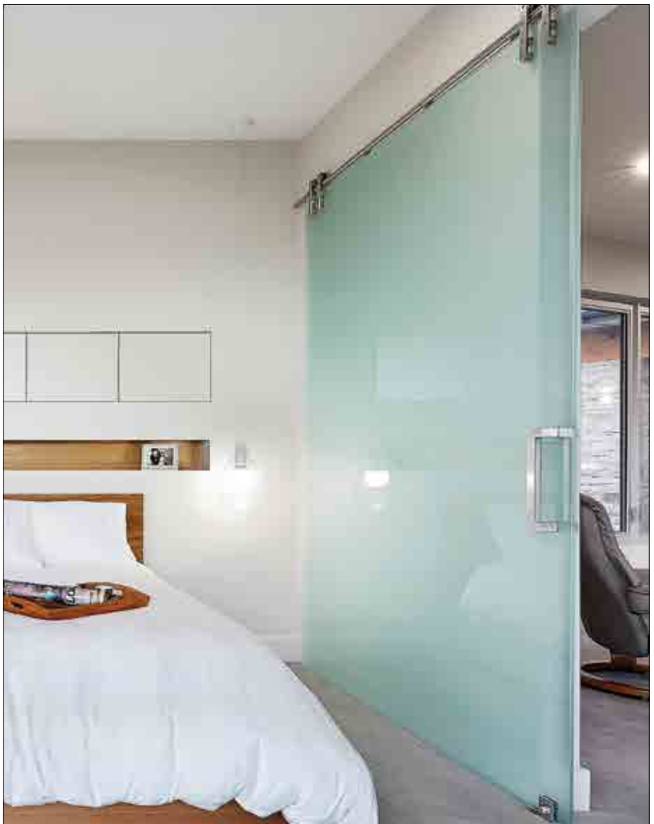
Figure 52 Glass Cut Outs Allow Affixed Hardware on an Internal Sliding Door
