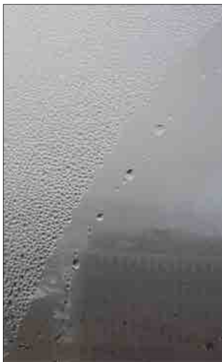
Figure 28 Condensation on a Window Source: Australian Window Association
