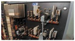
Electrical switchboard with asbestos flash guards. Switchboards can also contain an A-C sheet or resin/black backboard that contains asbestos. (non-friable)
