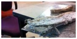
Mastic backed Asbestos fibre fire stopping around HVAC / other penetrations (friable)
