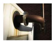
Asbestos gaskets in pipe flange joints (non-friable unless disturbed)
