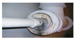
Amosite and chrysotile packing on a water pipe (friable)
