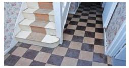
PVC or vinyl floor tiles and/or backing material with added asbestos (low %) chrysotile (non-friable). Tiles may also be laid on "black jack" adhesive containing chrysotile asbestos.
