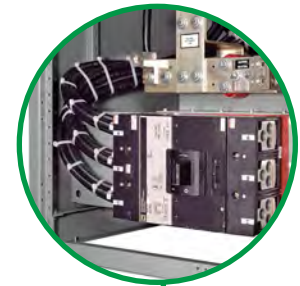
Fig. 13: Ground and neutral disconnect links
