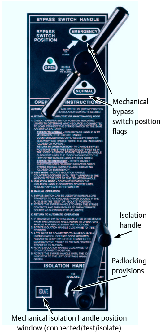
Fig. 12: Bypass-Isolation Switch user interface
