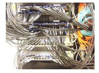
Fig. 8 Photo showing "cable sprawl" from networking equipment.
