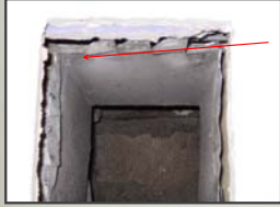
1. Termination point between horizontal runout of exhaust riser and sheetrock wall
