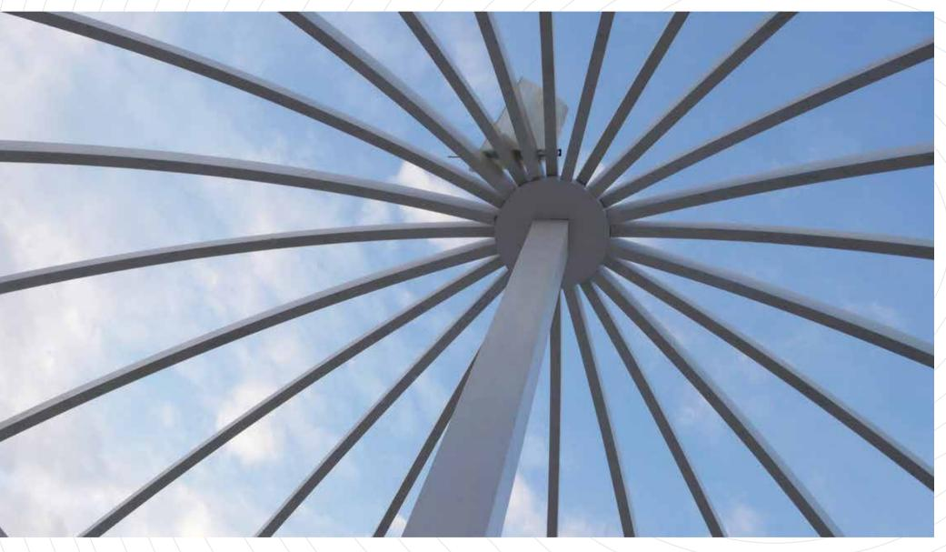
The structure having 12 m diameter is located on the terrace of Russia Federation Embassy -13storey building in the capital city Ashgabat. Without using a metal connection technology product, it was built with wooden dowels and interlocking system by forming radius timber truss. The dome that was the highest building of Ashgabat stands out with its location, architecture and construction technique.
