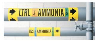
A uniform method of pipe identification, such as this one utilizing IIAR Pipe Markers, helps create a safer, more productive work environment.
