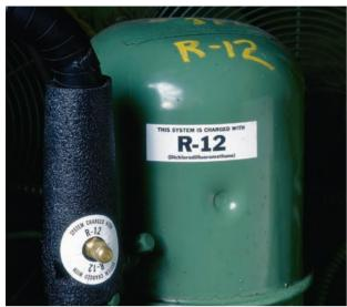
Markers such as these provide clear, professional refrigerant identification and eliminate the confusion and problems caused by charging a system with the wrong refrigerant.
