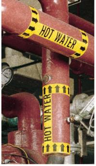
Secure Self-Sticking Vinyl Pipe Markers with Arrow Tape to identify flow direction and reinforce color coding.
