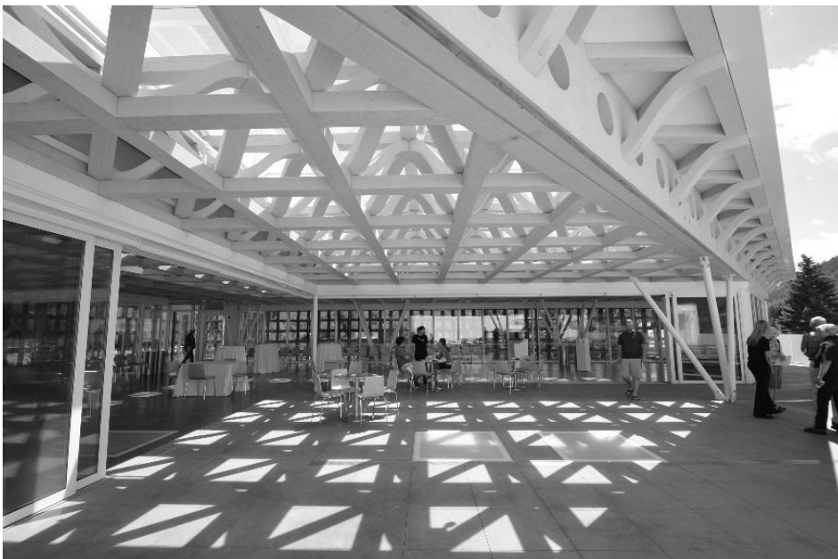
Figure 17: View of the finished truss on opening day - exterior
