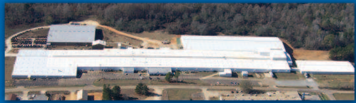
Nexans AmerCable's manufacturing facility in El Dorado, Arkansas.
