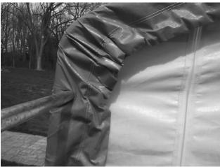
End Door Panels have pre-cut slots that allow frame members to pass through so rope pocket is inside unit.
