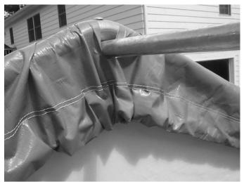
The rope channels should be located inside the unit, with the frame members passing through the pre-cut slots in the end panel/door. Replace and tighten the carriage bolts after putting the end panel into position.
