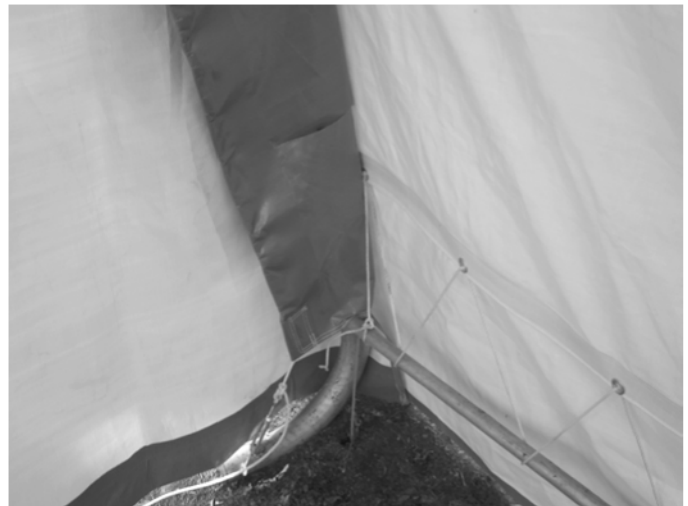
Inside Corner view showing Main Cover and End Panel Door properly laced and secured with turnbuckles.
