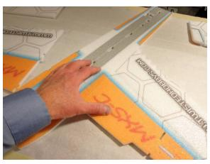
Once the glue has tacked up, carefully press wings back on for a permanent bond
