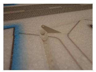
Glue aileron horns in. Make sure it is flush with the underside of the aileron and that the hole is in line with the pivot point. Cut the slot deeper if needed
