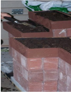
Figure 12. Green Roof Hardware Scale Model being built.
