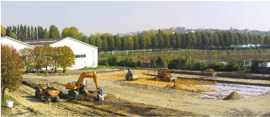
Figure 8 – The flexible pavement during construction (Photograph by M. Broutin)
