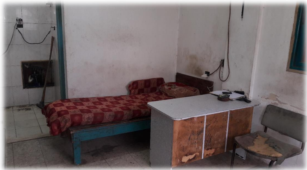
Figure( 3-8): Place were Workers Sleep During Duty in WWTP .
