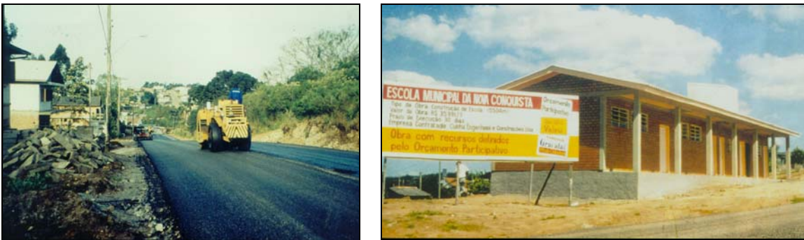
Projects developed with resources allocated by OP. Right: Caxias do Sul, Road Pavement. Left: Gravataí, School.
