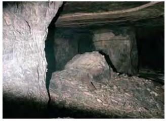
likely to be the lowest strength members of the pillars in a layout, and do not represent the average strength of the pillars. It was further observed that most of the failed pillars had been stable on initial mining but became unstable when the height was increased by floor benching.
