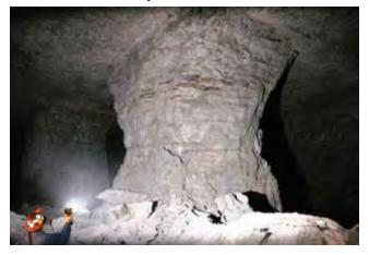
splitting parallel to the applied load in low confinement (Diederichs, 2002). Splitting and slabbing of limestone was observed at stress levels that are only less than 12 percent of the UCS of the rock (Iannacchione, 1999), which indicates that pillar strength might be significantly reduced in the absence of confinement.
