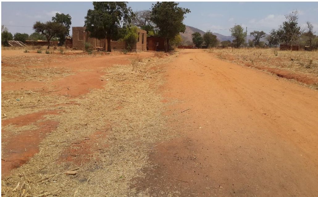
Figure 4.9: The rehabilitated road in Sokoni - Ukalanza in Chamwino
