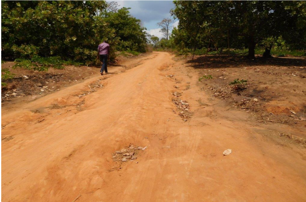
Figure 4.8: 5-km feeder road constructed in Mkongi, Lindi D.C.
