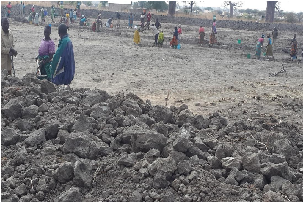
Figure 4.5: Actual rehabilitation works of charco dam in Chinangali II village (Chamwino)
