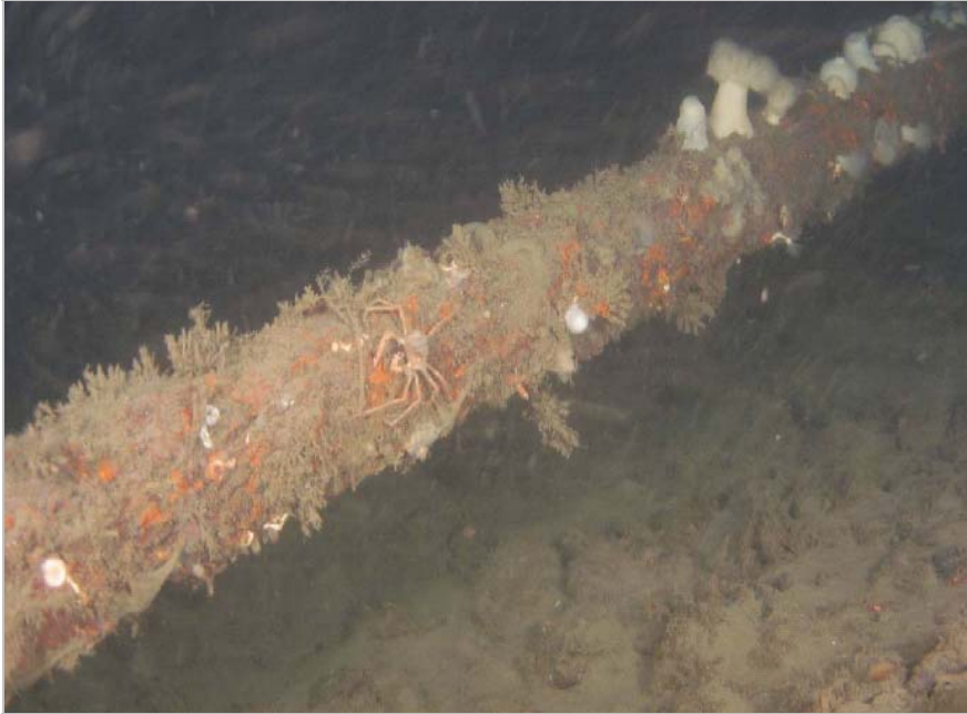
Figure 1: Sub-sea cable, in place for approximately 50 years, covered with sessile encrusting organisms at Vancouver Island (BCTC, 2006).
