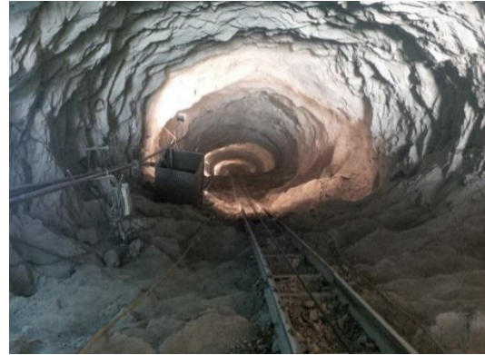
Picture 2 Excavated view of the escape tunnel and rail track
