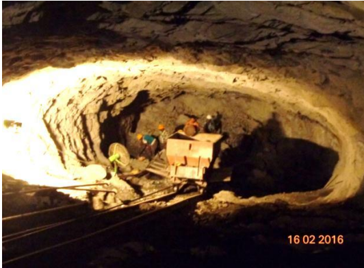
Picture 1 Manual mucking with bucket/trolley using rail track
