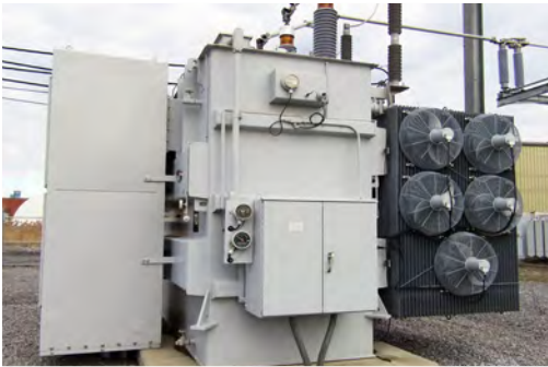
2015 ABB 30MVA POWER TRANSFORMER
