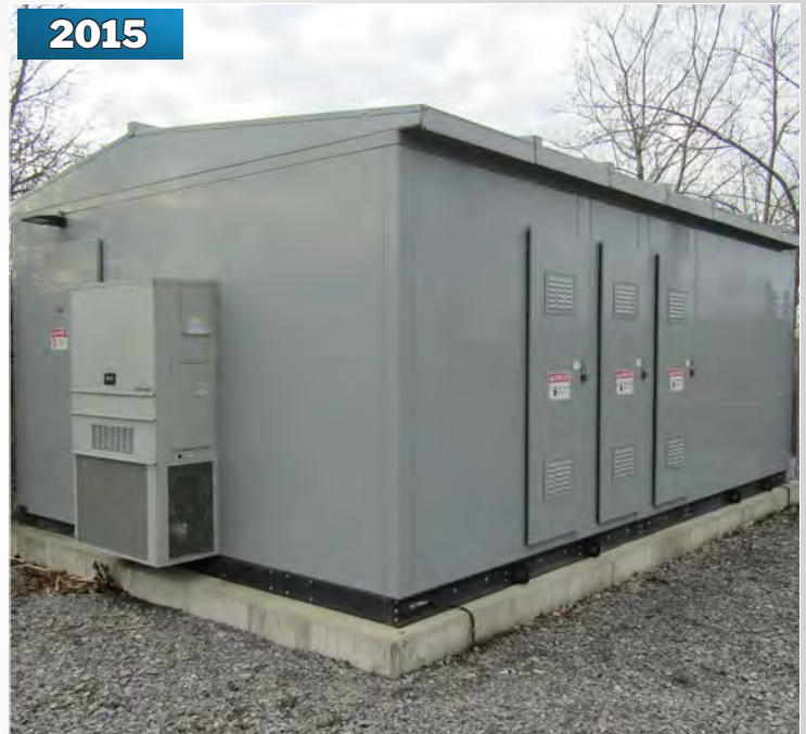
ABB 15KV, 2000AMP METAL-CLAD OUTDOOR SWITCHGEAR ASSEMBLY BY JAGG
