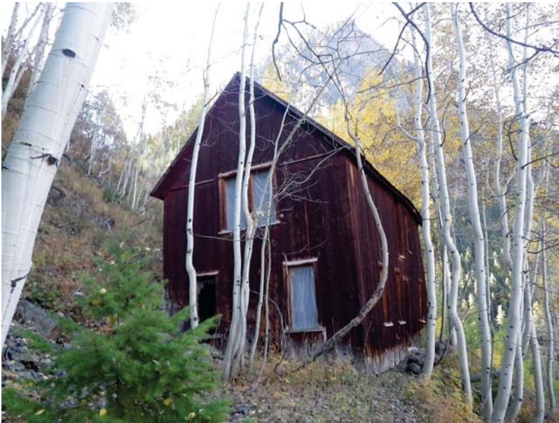
Photo 7. Looking W at old Thistledown bunkhouse located upslope from Disposal Parcel C on Rockbiter-owned land (Argyle Claim).
