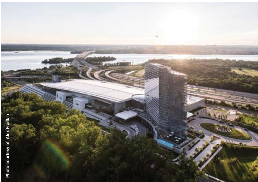
Precast concrete profiles and panels clad the plinth, a stepped structure housing the parking garage.
