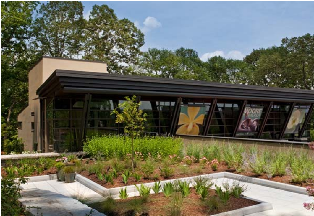
Figure 3 Green Roof covering a part of the Hardin Visitor Center
