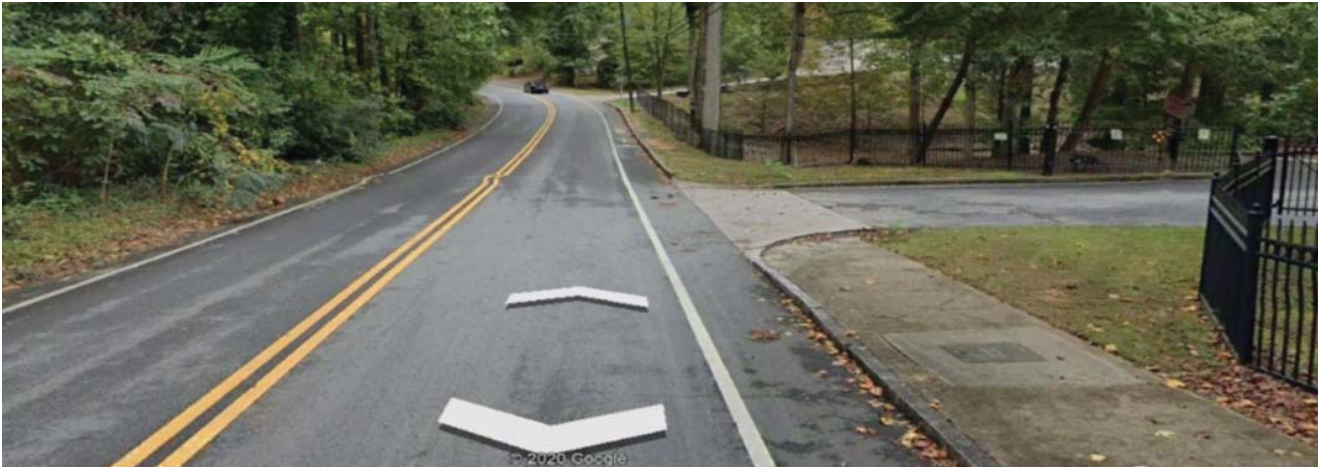
Figure 5 - Google Earth image showing current sidewalk ending on Collier Road at church entry, sidewalk infrastructure should extend farther beyond to assist pedestrians in safe passage.
