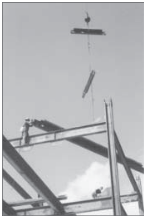
Ironworkers prepare to connect a steel beam.
