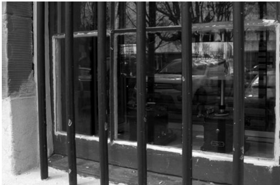
Figure 66: Salamanca Place: insert time , 2010, exterior view
