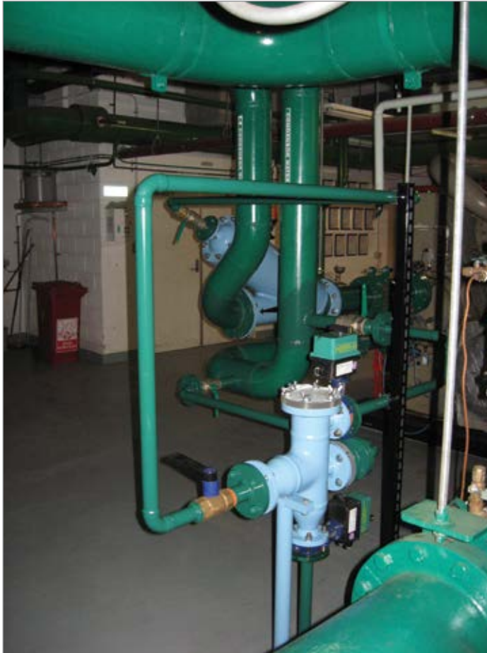
Figure 5: The sponge ball ATCS installed in Case 1
