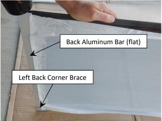
5. Install the Rafter with the Left Back Corner Brace on the PC Sheet, then drive in the Back Aluminum Bar using a rubber mallet.
