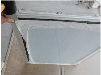
8. Install the Front Aluminum Bar with the two Braces onto the PC Sheet.
