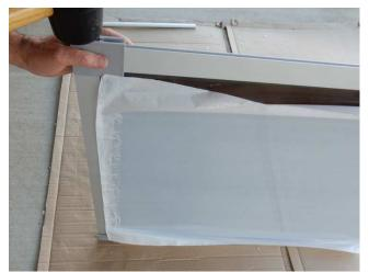
6. Install the Rafter with the Back Connector Brace.
