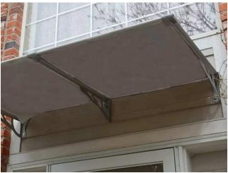
15. Attach the Extension Unit to the Main Unit and secure to the wall using appropriate wall anchors.
