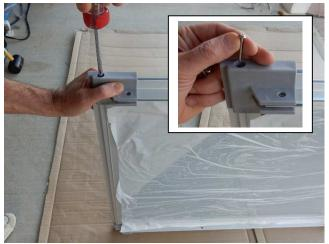
9. Drive a Small Screw into both ends of the Back and Front Aluminum Bars through the holes in the Corner Braces and Connector Braces.
