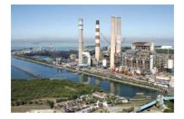
The station operates four (4) pulverized coal-fired steam units equipped with desulfurization scrubbers, electrostatic precipitators, and selective catalytic reduction (SCR) air pollution control systems. In addition, the station operates one (1) aeroderivative combustion turbine that entered into service in 2009 and can be fired with natural gas or distillate oil.
