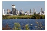
The station operates five (5) generating units. Polk Unit 1 is an integrated gasification combined cycle (IGCC) unit fired with synthetic gas produced from gasified coal and other carbonaceous fuels. This technology integrates state-of-the-art environmental processes to create a clean fuel gas from a variety of feedstock with the efficiency benefits of combined cycle generation equipment. Polk Units 2 through 5 are combustion turbines fired
