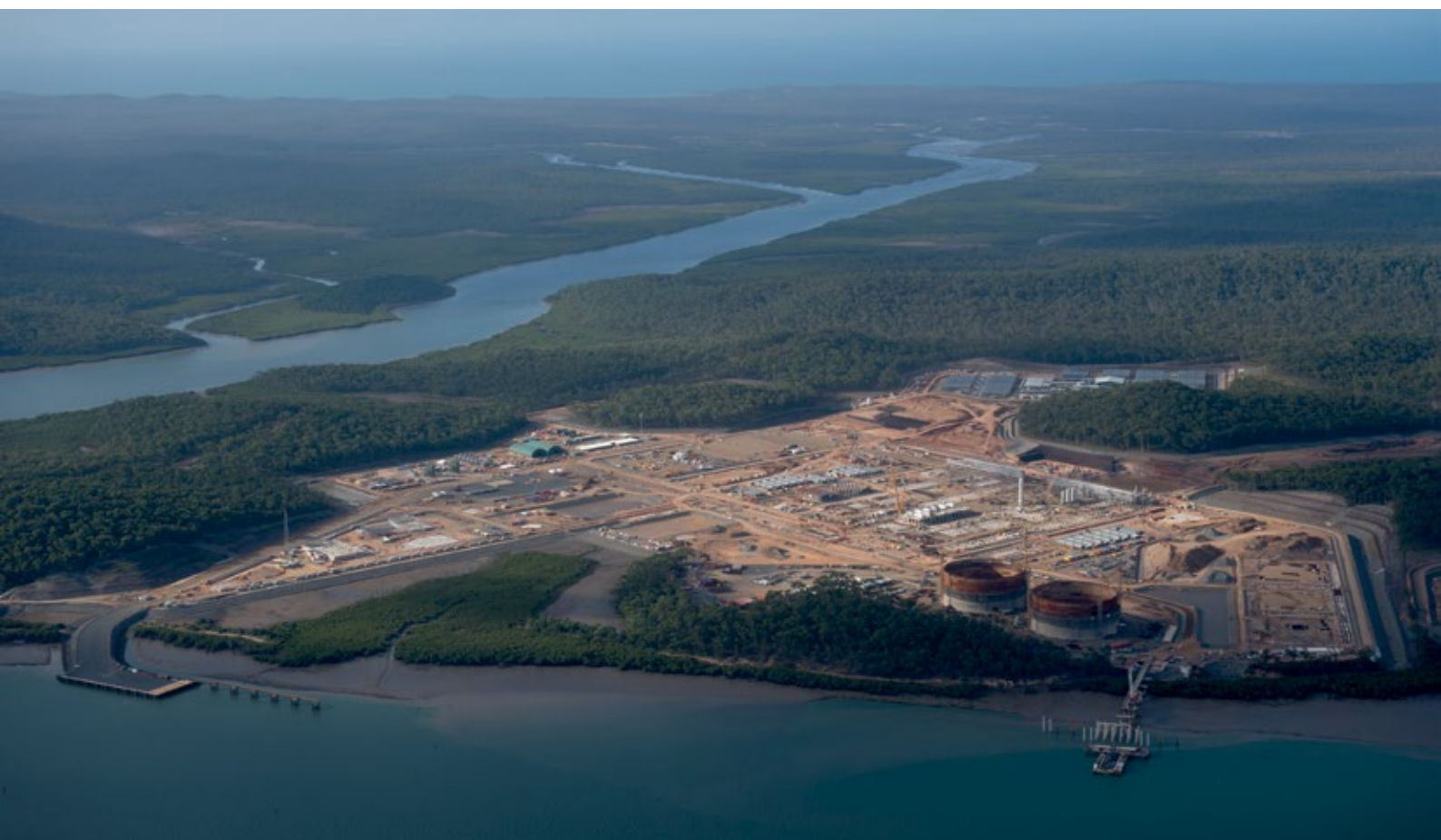
Figure 9: Stationary energy emissions have been increasing over the past decade largely as a result of increasing LNG production (pictured) and mining operations.
