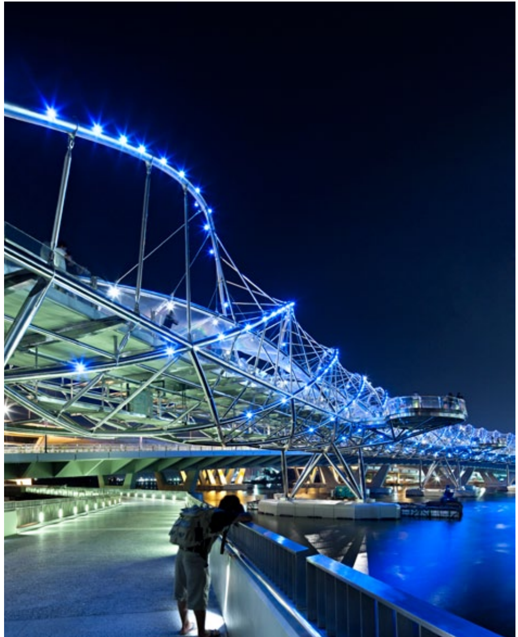
▲ Helix Bridge, Singapore
