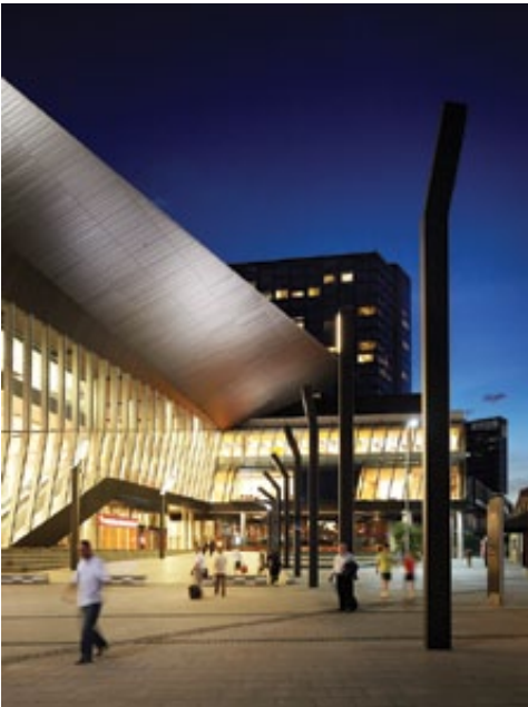
▲ Melbourne Convention Centre, VIC, Australia 6 Star Green Star – Convention Centre Design PILOT
