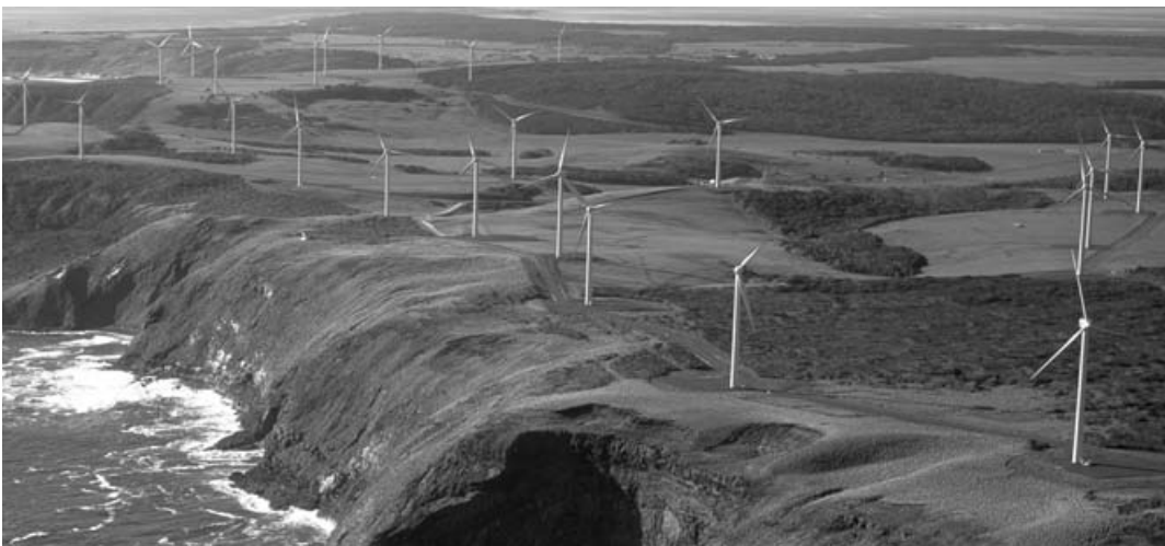
Woolnorth Wind Farm. Source: Hydro Tasmania
