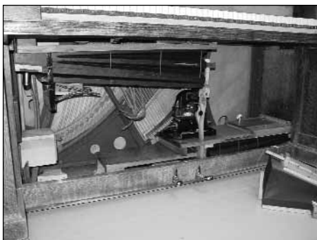
The restored pumps and gear standard installed, vacuum reservoir ready to be installed.
