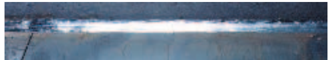
Figure 4. Bead appearance. The standing fillet weld is flat with a smooth blending of the toes.
