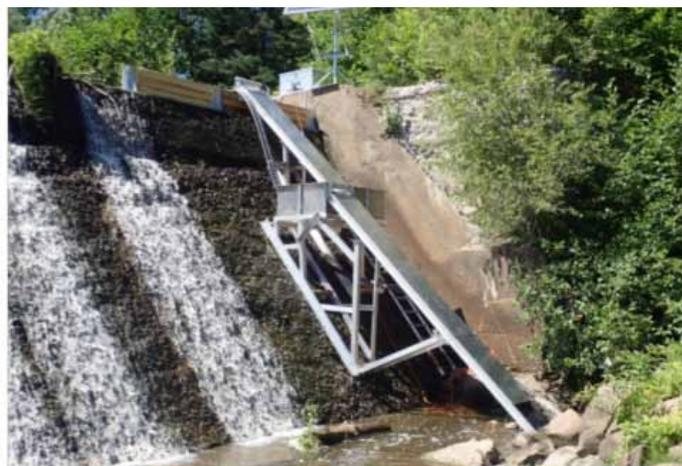
Figure 1: Ladder for eels set up in the watershed of the Portneuf River
