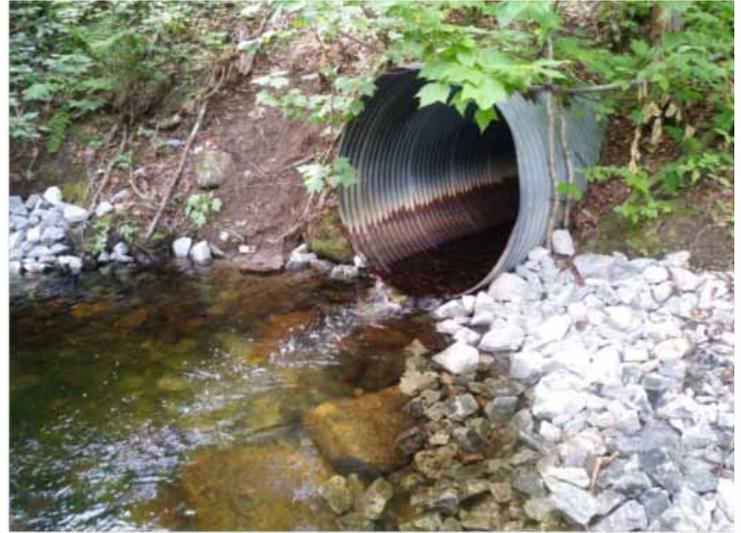
Figure 3: Upgrading of a pipe downstream of a culvert on the Éternité River allowing access to the American eel. Photo: Akian Gros-Louis Picard
