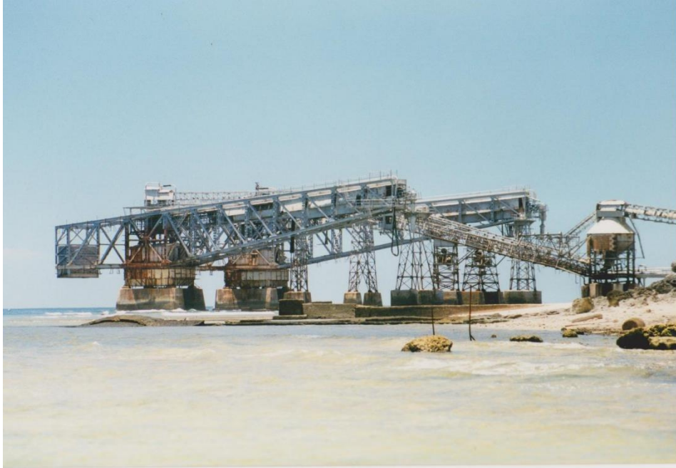
Phosphate loading cantilevers – destroyed reef
