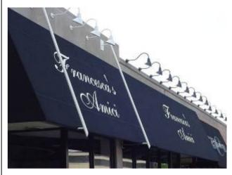
Gooseneck fixtures spaced too close together and too many in a row(4d)
