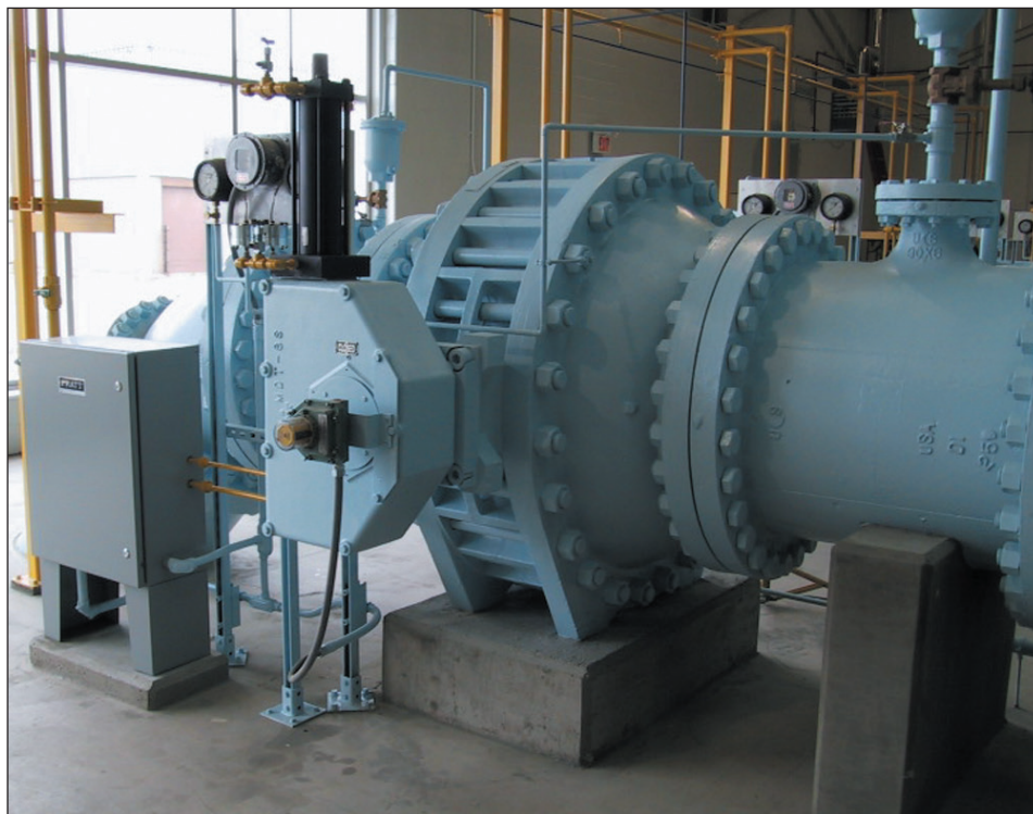
Rubber Seated Ball Valve Installation
