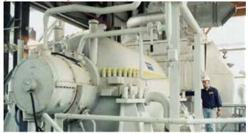
**Barrel** – Vertically-split barrel compressors are used primarily for high-pressure applications such as ammonia, urea and methanol synthesis, refinery recycle, natural gas compression and injection, and hazardous gases.
