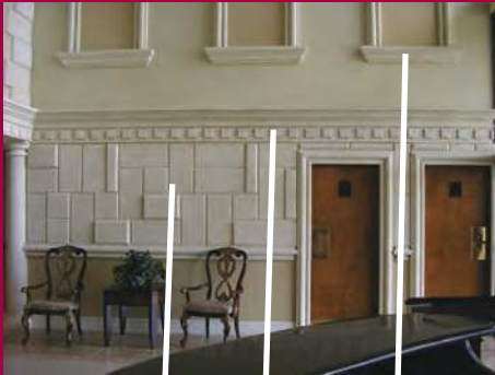
Wall Treatment, Molding and Sills
