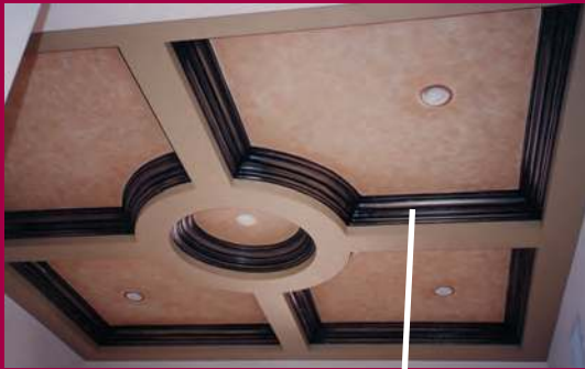
Tray Ceiling with Molding
