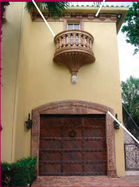
Window Balcony w/Balusters & Brackets under eave
