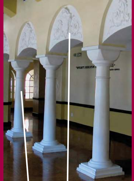
Columns and Arches with Appliques
