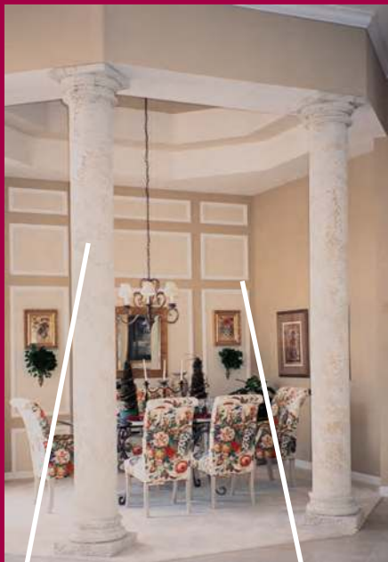
Columns with Caps and Bases and Wall Molding
