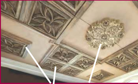
Ceiling Tiles and Medallion
