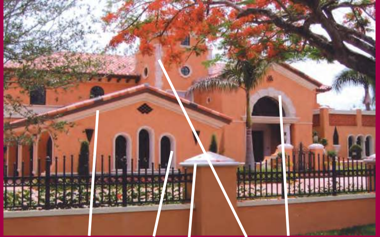
Molding, Arch Windows, Wall Caps, Quoins and Arch
