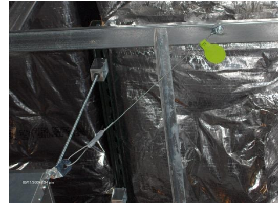
DUCTWORK SEISMIC RESTRAINT DETAILS
