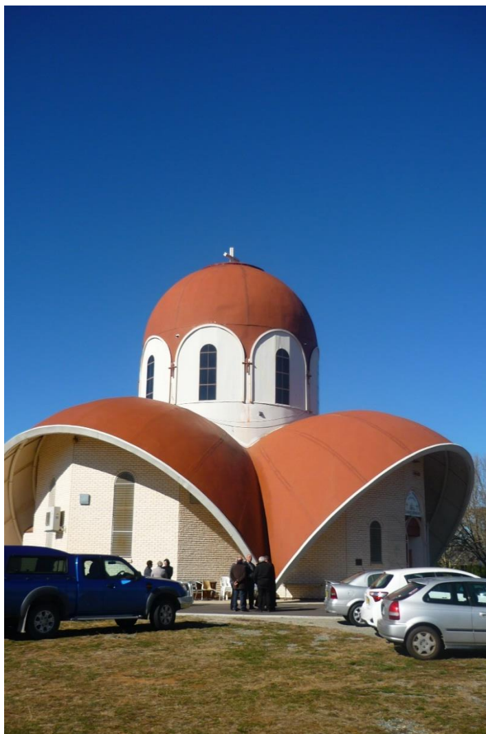
Image 2: This photo shows the exterior of the Church from the front access road off Goyder Street (ACT Heritage 2019)
