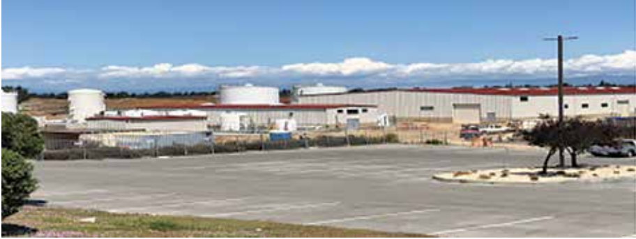
The newly completed Pure Water Monterey water recycling plant.
