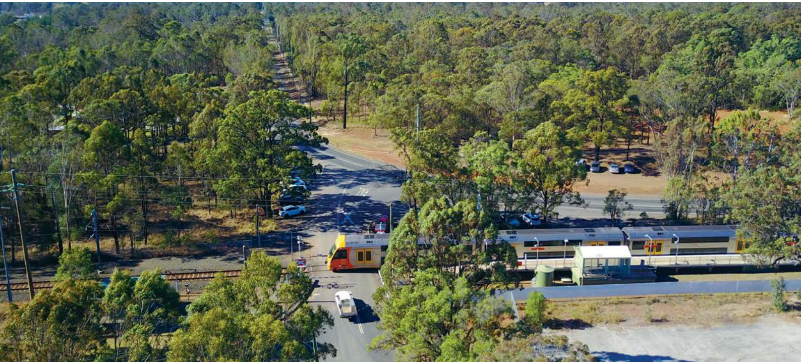
Aerial of Bandon Road and Vineyard Station facing east
