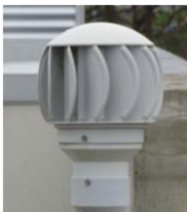
Figure 1. Wind turbine ventilator (Sewer vent)
